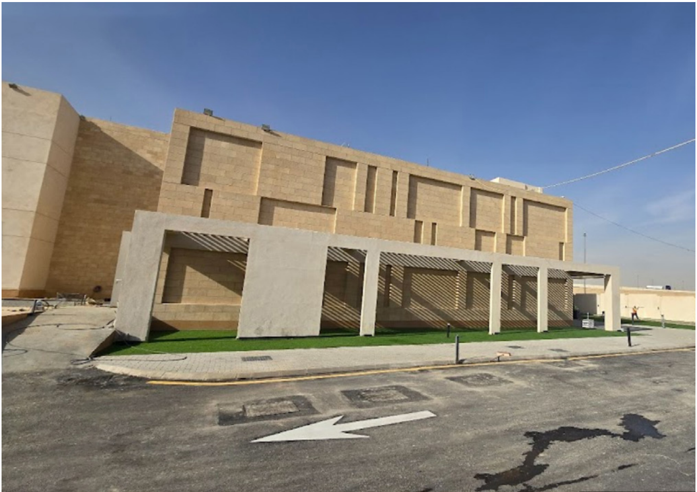
MOBILY DATA CENTER
