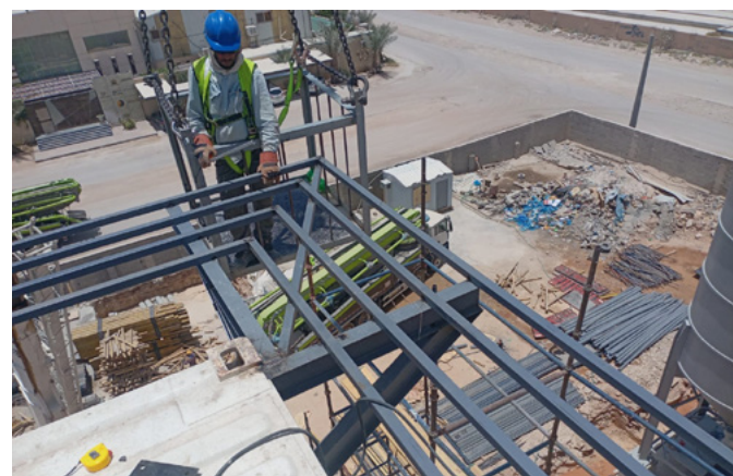
MIX STEEL FABRICATION PROJECT
