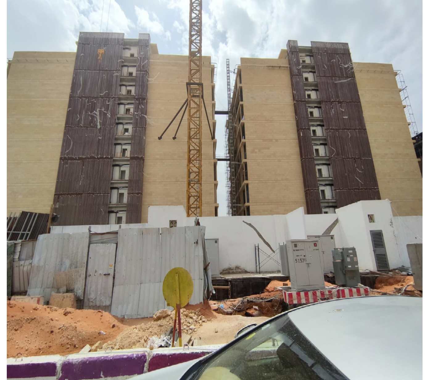
Summod Tower Project
